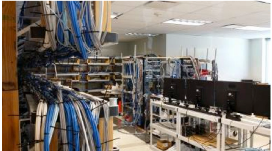
Figure 2. Overview of test setup showing bundled cabling connecting HDBaseT transmitter and receiver equipment
